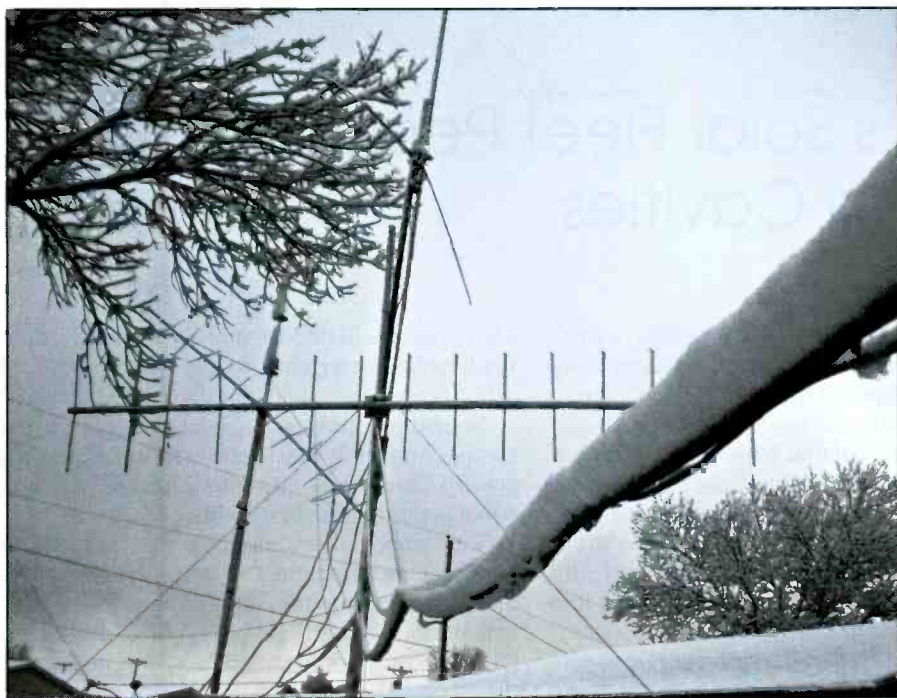
Photo E. Nestled in Mike Coletta's monitoring station antenna farm is a vertically-polarized 15-element Yagi used for aviation monitoring.
